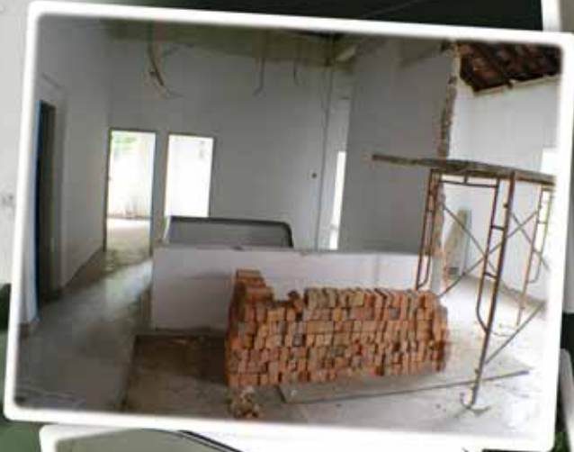
Airy and spacious former dormitory rooms are partitioned for office spaces
