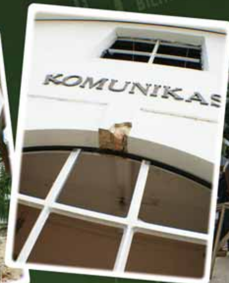
A damaged crucial portion of an arch
