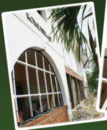
An arch being bricked up into a window
