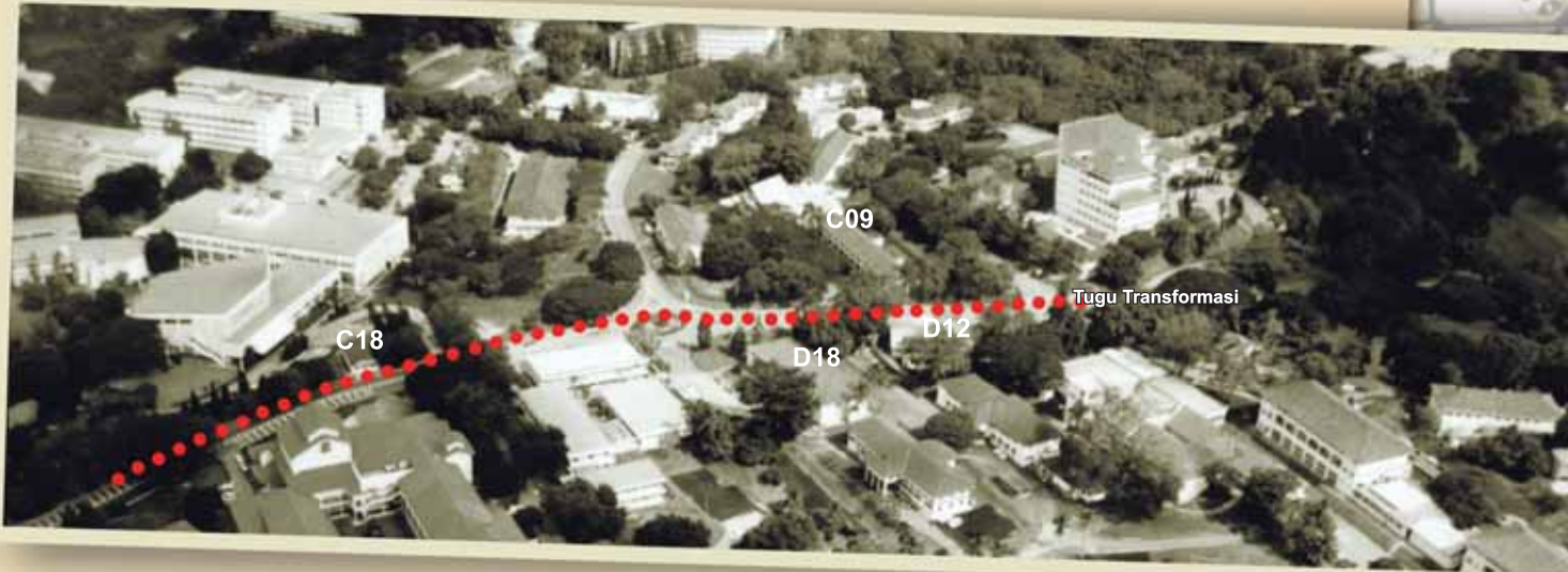
The high street (dotted in red) in the 1990's (Photograph courtesy of Pusat Teknologi Pengajaran dan Multimedia, USM)
