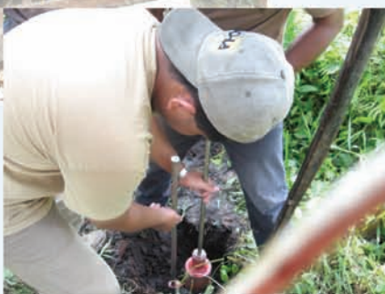
Conducting soil test before the reconstruction of a school
