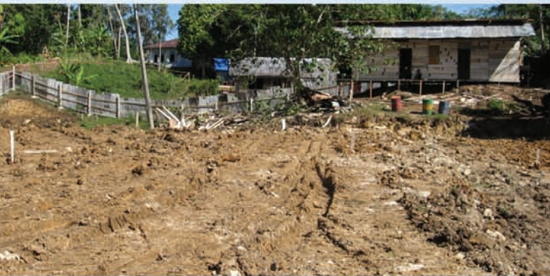
Site preparation for a school in Sisobahili Tabaloho Dahan, Nias Island
