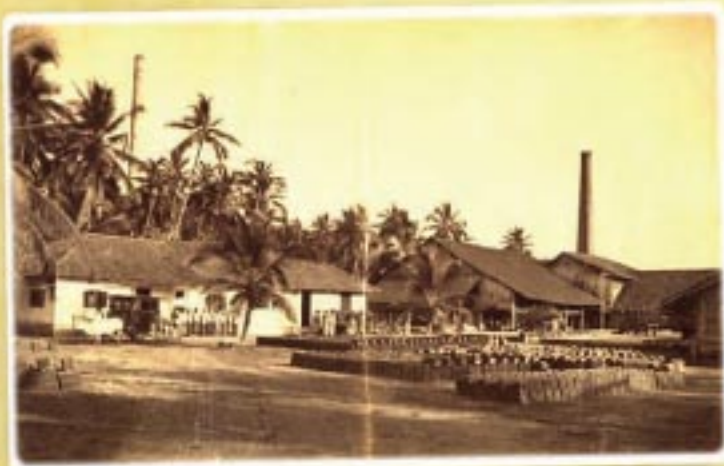
Basel Mission Tile Factory on the bank of Nethravathi River (Source: Basel Mission Archive-Mission 21 )
